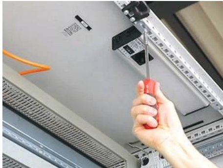
Assembly with screws on surfaces
