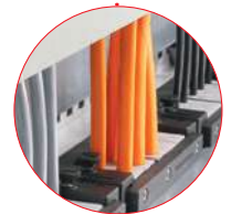
Straight cable routing into the cable duct
