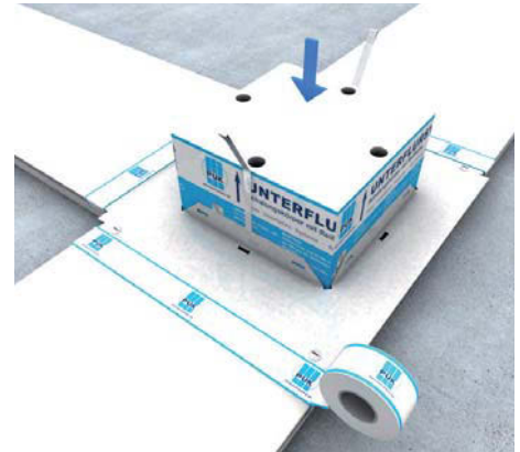
12 | Shuttering unit Insert shuttering unit straight, arrow pointing up, into the opening of the assembly cover. All open areas must be masked according to DIN before applying the screed.
